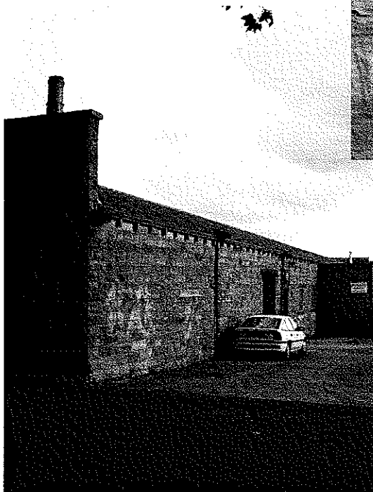
Queen Street Mill elevation to the site
