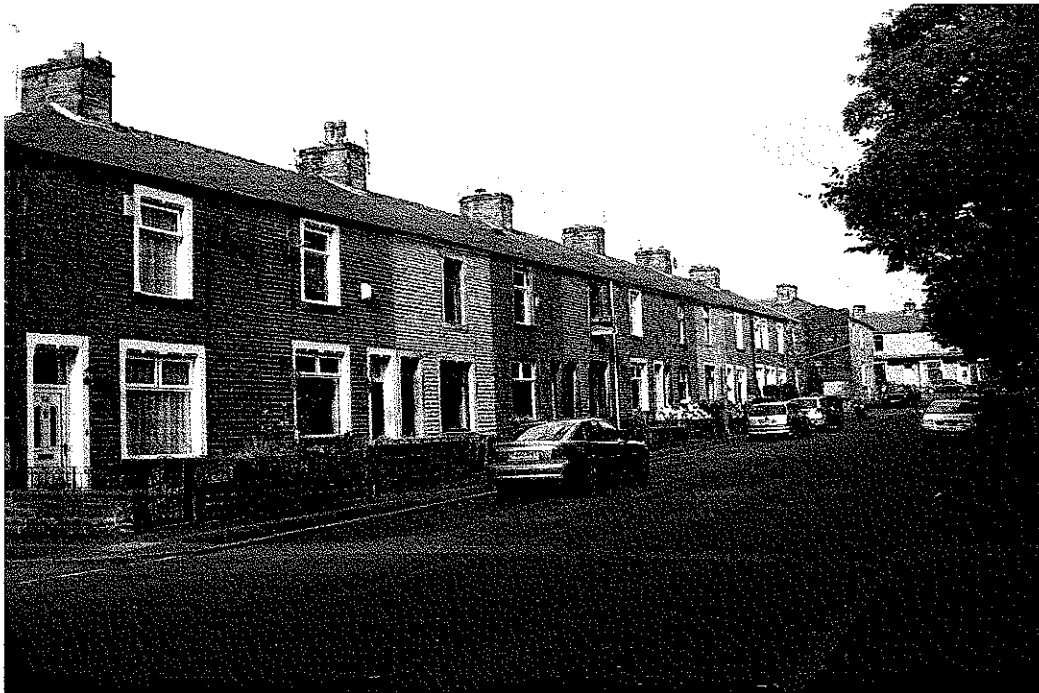
Existing streetscape to Church Street
