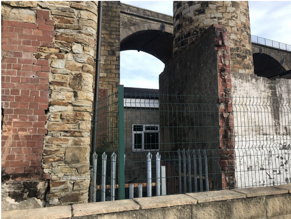
View of yard area partially demolished
