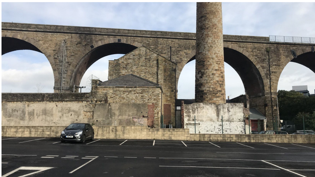
View Looking North Towards Ashfield Mill Engine House
