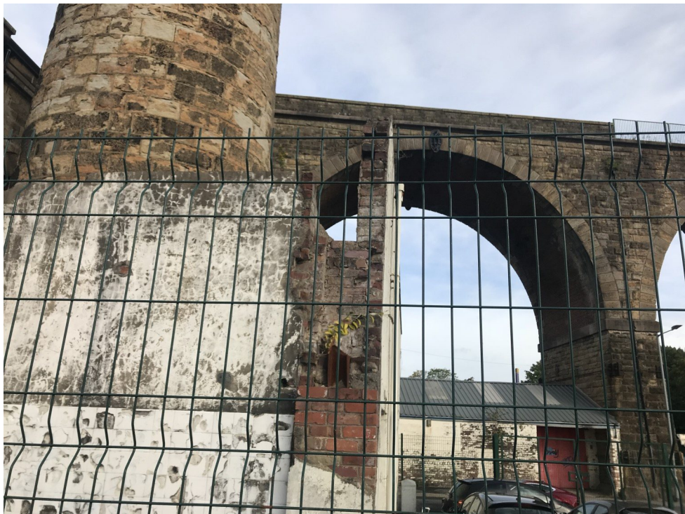
View of Chimney Base
