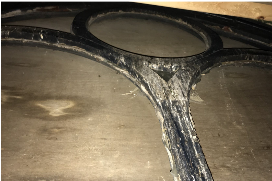
Existing circular wooden tracery inside view
