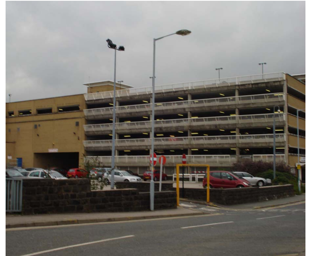
Fig 2.4.3 Royle Road and Millennium car park
