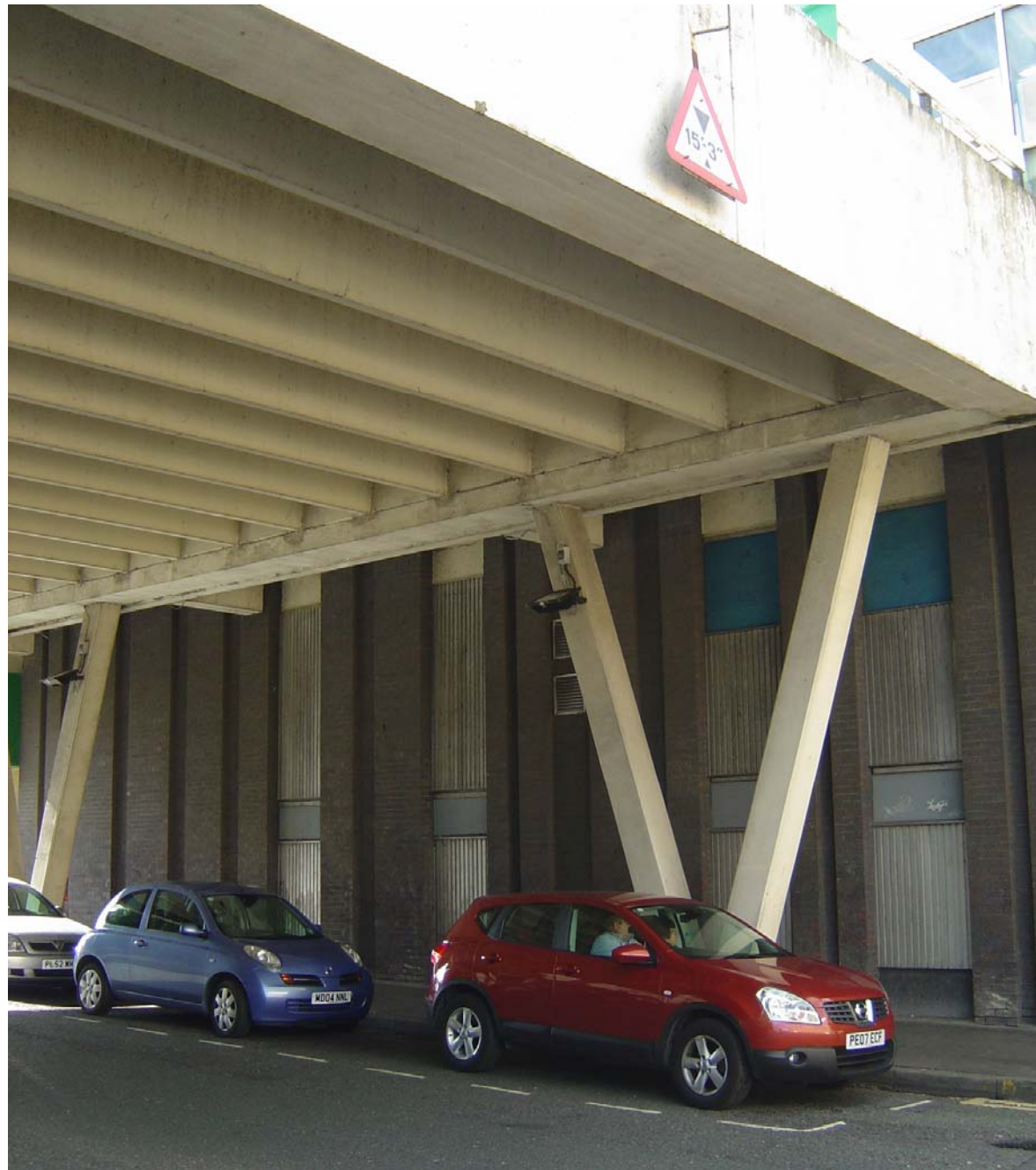
Fig 2.5.4 Existing market hall complex high level platform & Bankfield beneath
