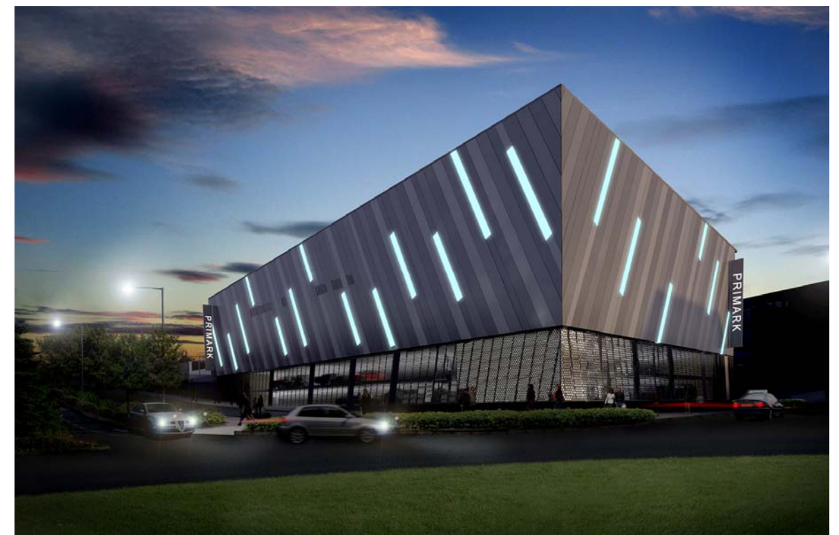
Fig 6.5.2.11 View from Active Way by night, looking towards unit 6 and the under-croft car park
