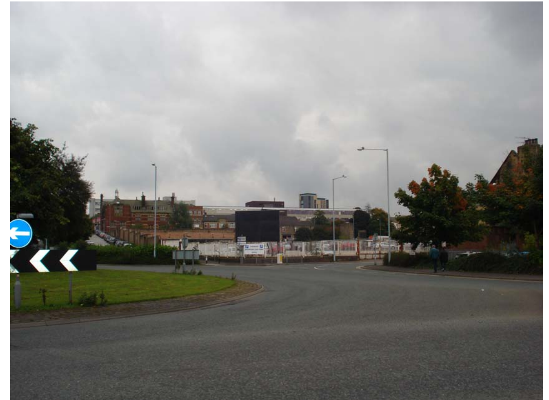
Fig 2.4.4.3 Active Way / Royle Road roundabout (development site to centre)
