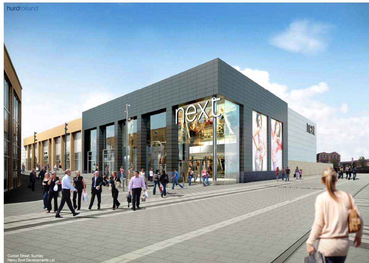
Fig 6.5.3.4 View from Curzon Street / Parker Street junction (unit 14 to left, unit 2 to right)
