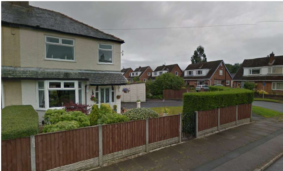
Frontage to Springwood Road
